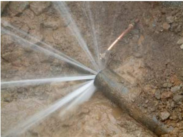
Fig. 1: A damaged pipeline
